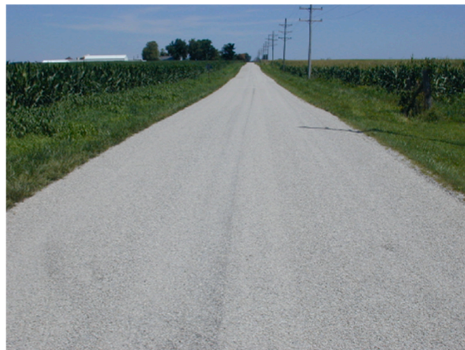
Fig. 4. Newly finished chip seal impervious roadway.
